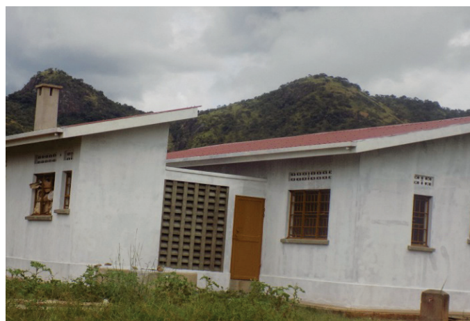
Newly constructed staff house in Alerek HC III
