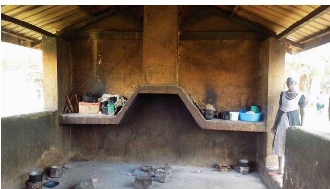
Kitchen in Abim General Hospital
