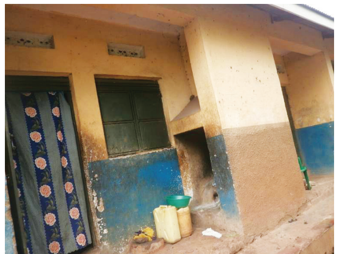
Staff Quarters in Nyakwae HC III
