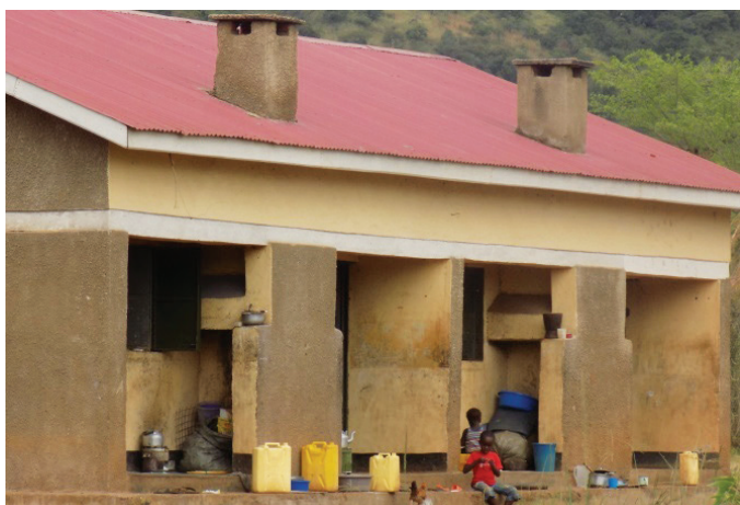
Staff house in Alerek HC III
