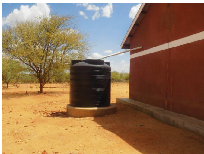
Water harvest tank in Alakas HC II
