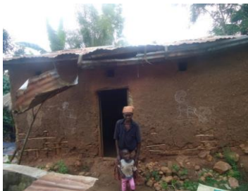
House and pit latrine before intervention
