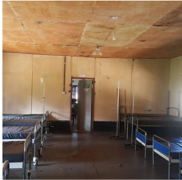
Maternity ward in Nakapiripirit HC III
