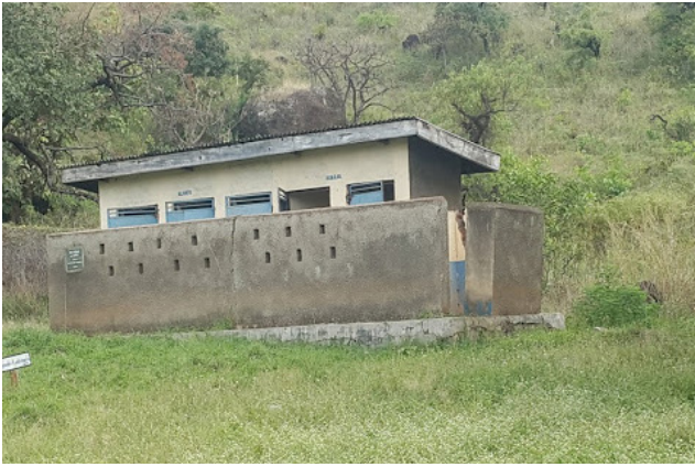
Latrine in Namalu HC III
