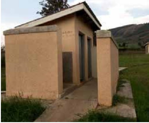
Toilets at kikagate HCIII
