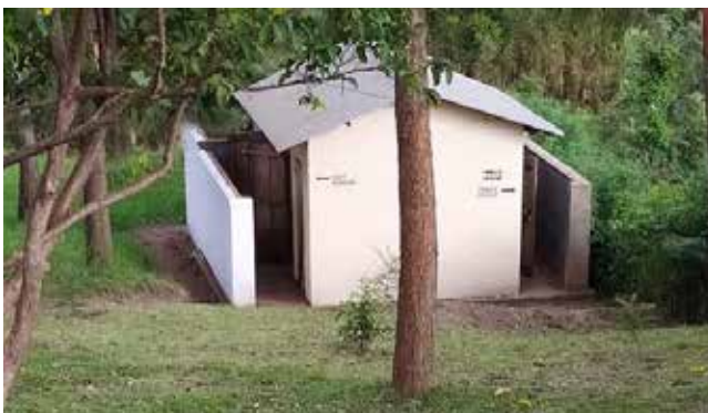
Toilet at Kakoma H/C III
