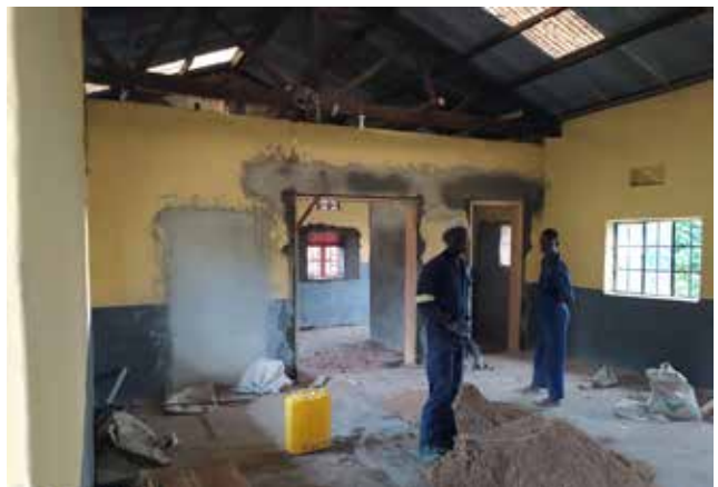
Repairs at Ngarama HCIII
