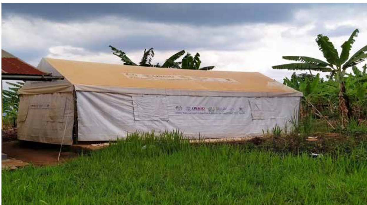
Tent at Ngarama HCIII, donated by RHITES SW for PLHIV to receive ART, strategically facing off the road to minimize stigma
