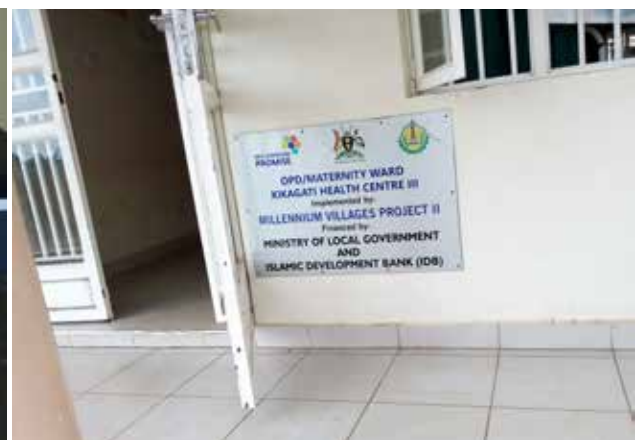
Newly constructed Maternity ward at Kikagate HCIII
