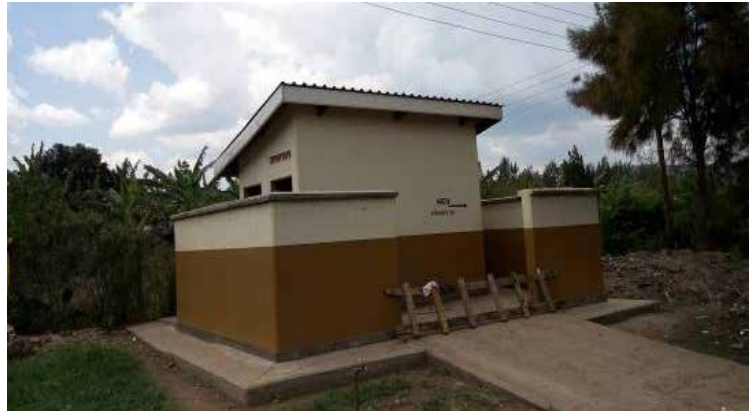
Toilet at Kabuyanda HCIV
