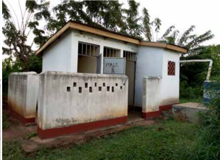
Toilets at Balawoli HCIII
