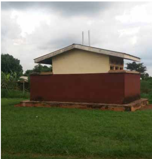
Toilet at Kitayunjwa H/C
