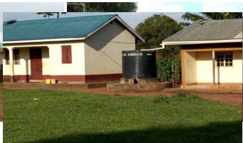
Rainwater harvesting at Balawoli HCIII
