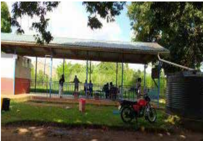
Shelter at Namwendwa HCIV
