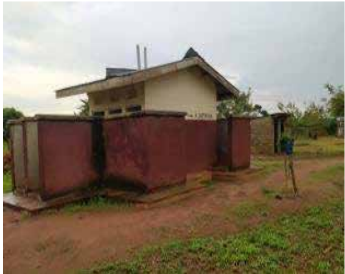
Toilet at Mbulamuti H/C III
