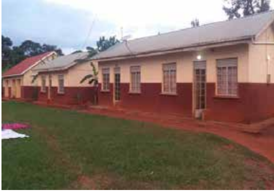
Staff quarters at Kitayunjwa HC III
