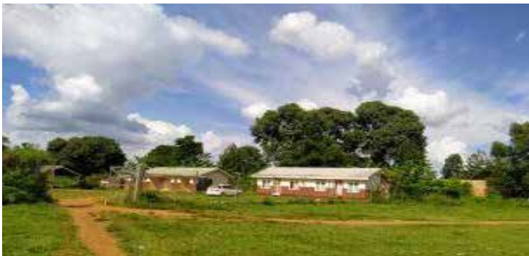
Namwendwa HCIV staff quarters (at maternity and theatre area)
