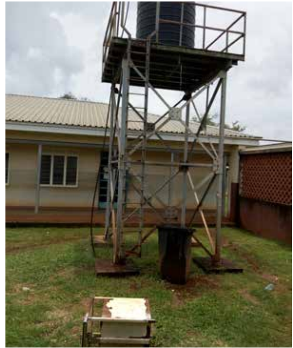
Kamuli GH water tank
